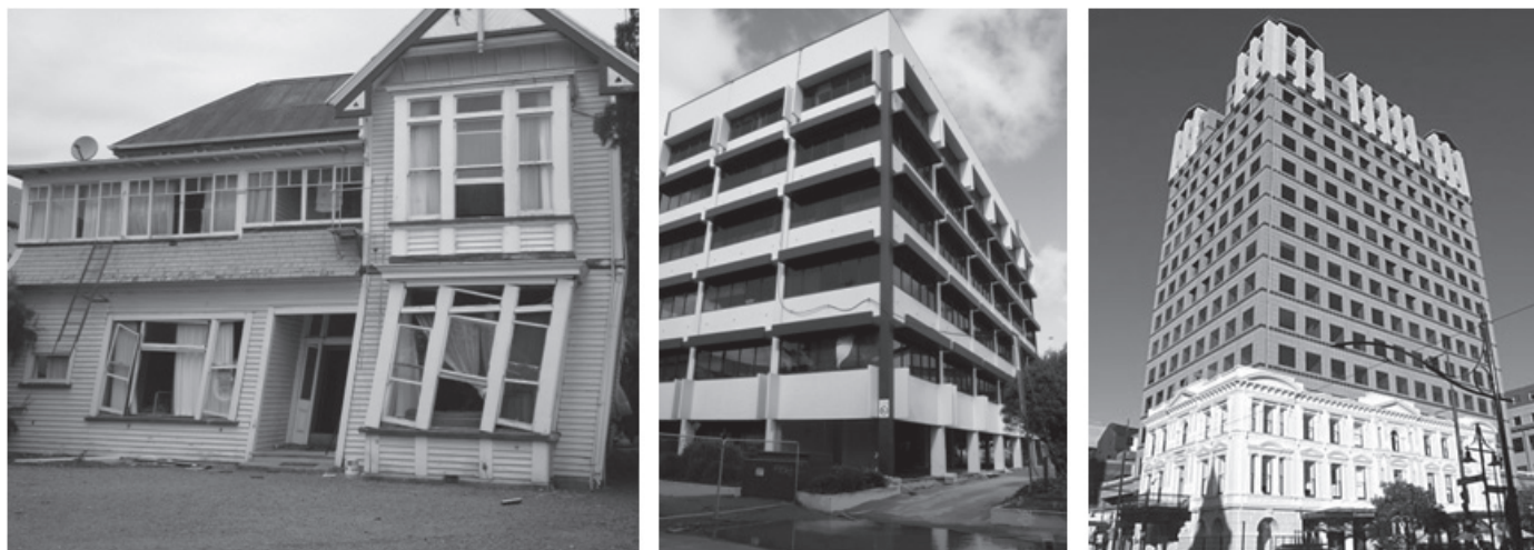
▲ Figure 9. Representative buildings for the considered categories: timber residential house (left), mid-rise RC structure (middle), and tall RC structure (right).
